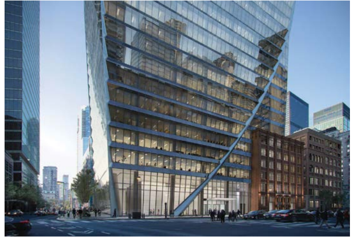
160 Front Street , a fully leased 1.3 million square foot office tower, is under construction and designed to achieve LEED Platinum and WELL certifications
